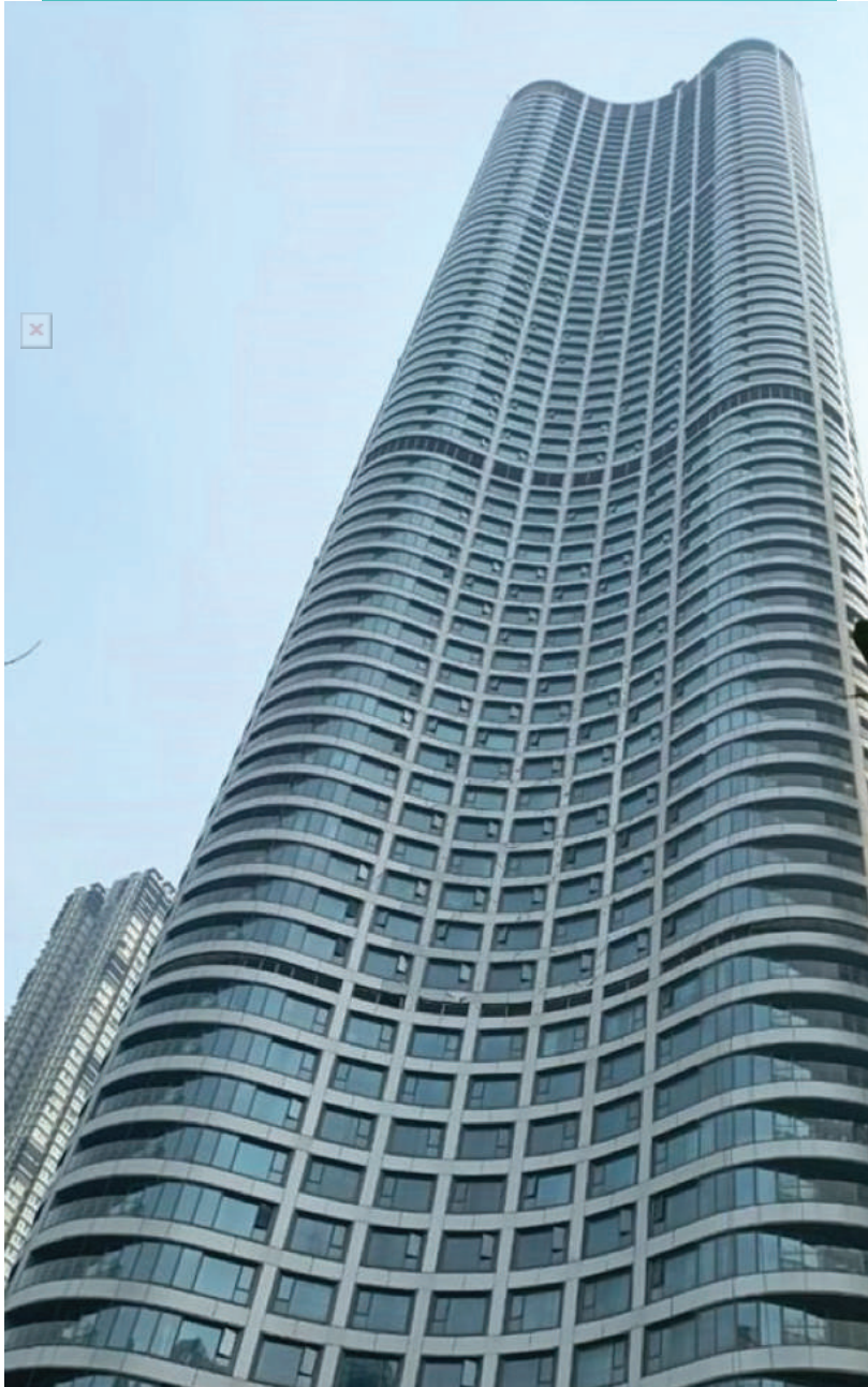
8 - Lodha World View (Residential - Window Work)
