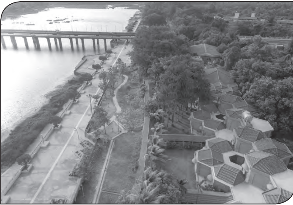
RAS BY TREAT-AERIAL VIEW
