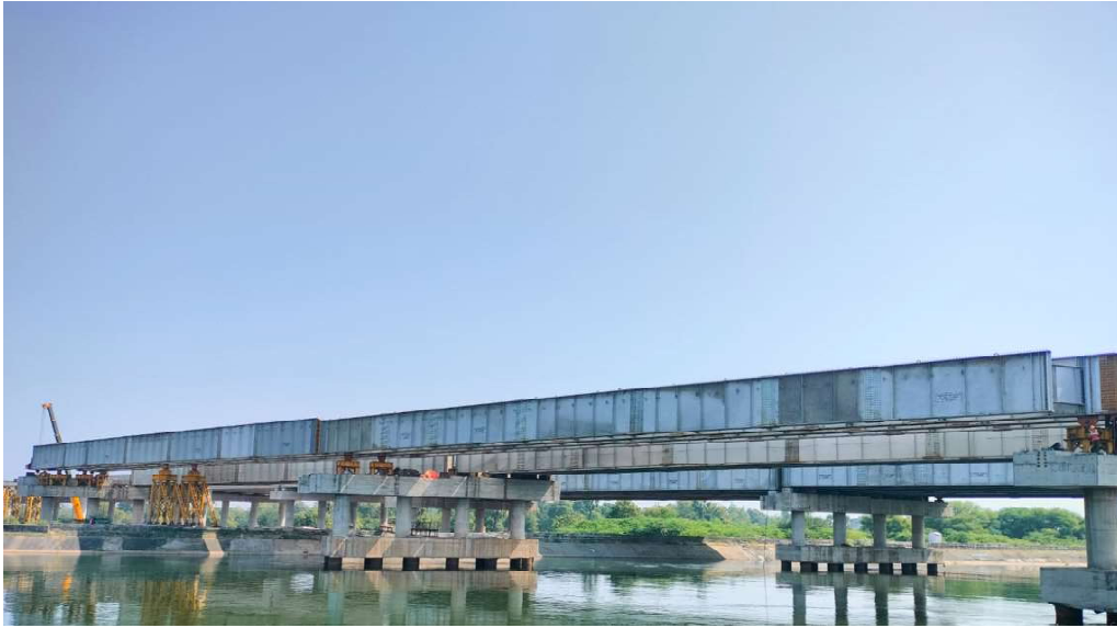
Eight Lane across Panchmahal Vadodara Gujarat
